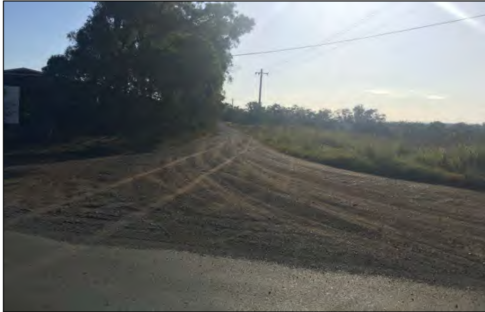
Figure 4: Sargents Road facing North East
