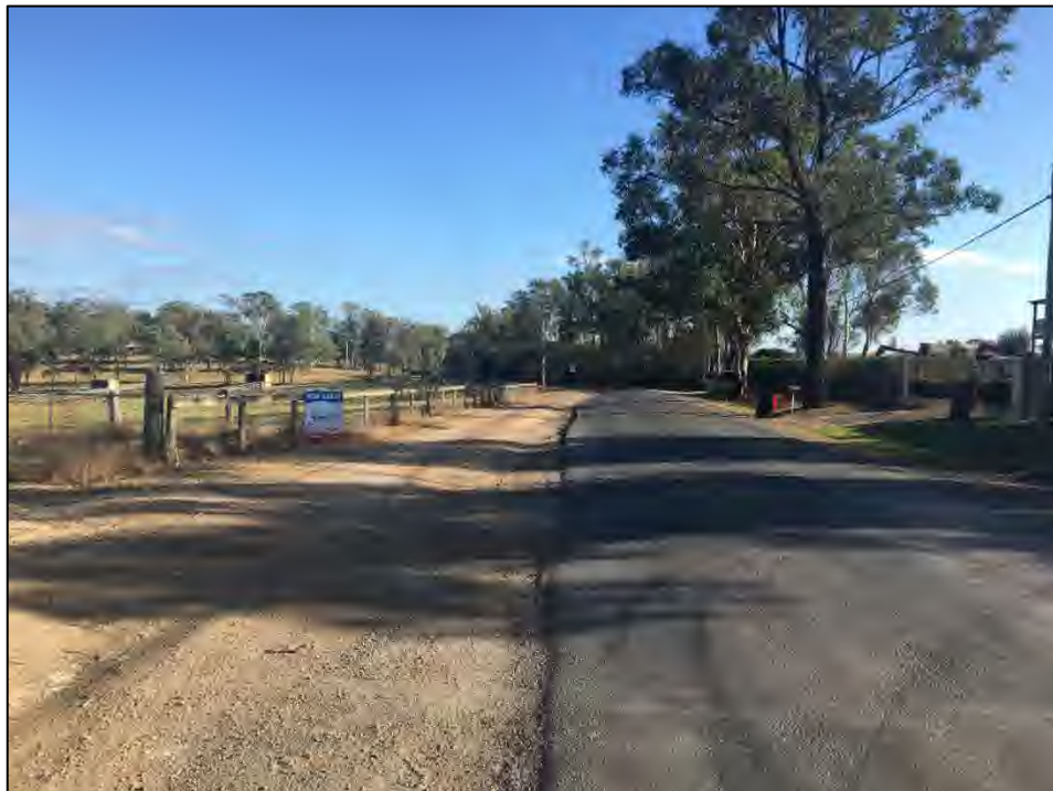
Figure 5: Stannix Park Road facing North West
