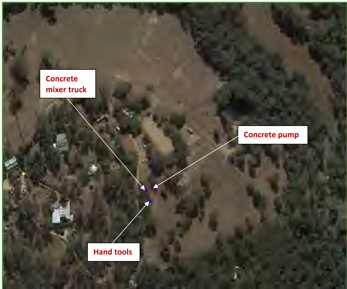
Figure 9-2: Construction Stage 2 – Concreting Construction Works
